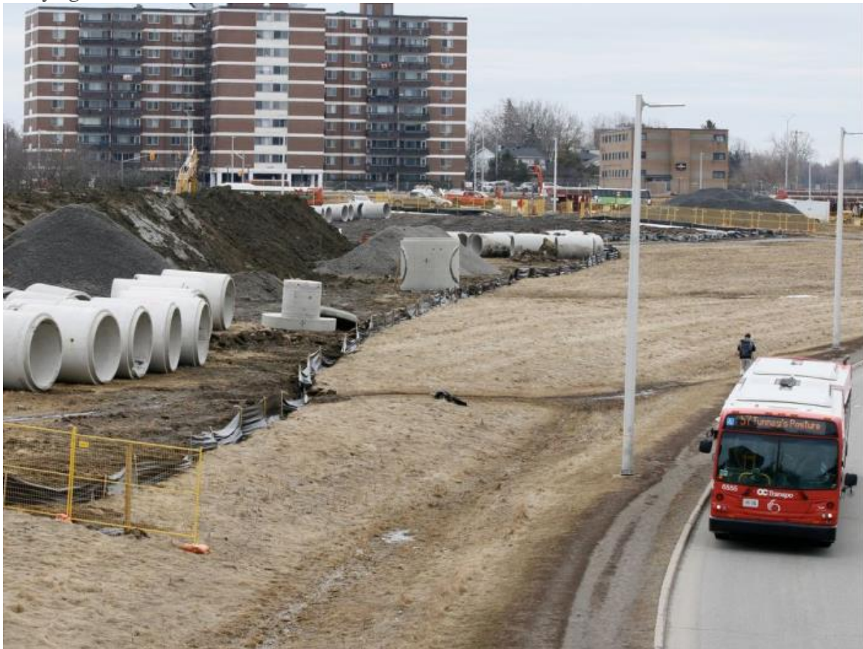
Stage 2 LRT construction near Lincoln Fields station. ERROL MCGIHON / Errol McGihon
